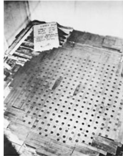
The “atomic pile” in which Enrico Fermi and Leo Szilard creating the first self-sustaining neutron chain reaction.
